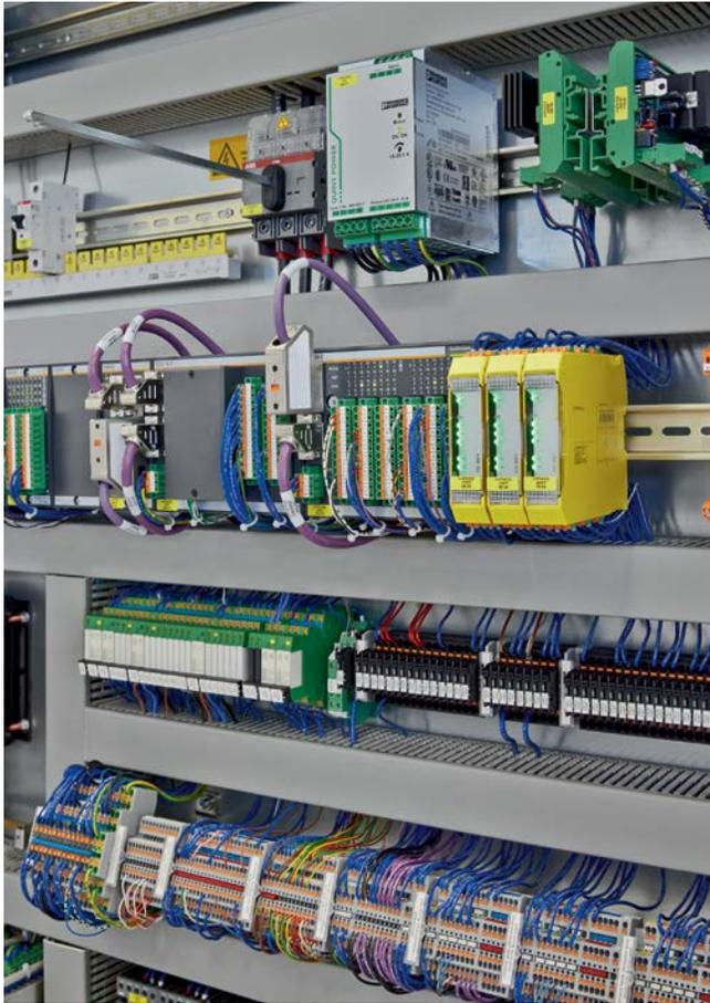
**Figure 1:** To automate its new selective-soldering systems, Ersä relies on multifunctional safety relays, as well as many additional components from Phoenix Contact.
